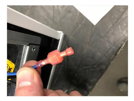
4. Locate the Yellow wire installed on the 24 volt (power) side of the transformer. Note: The terminal connector plugged into the transformer has a ¼" male spade available to install another terminal connector.
