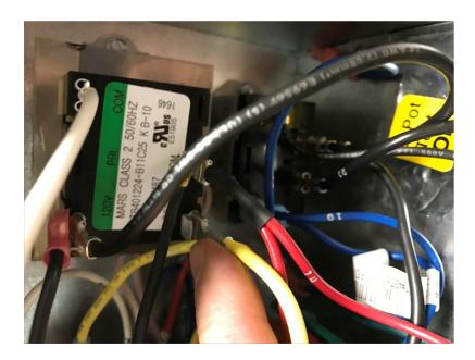
5. Using the new black wire provided in the rewire kit, install the ¼" female connector (with piggy-back male connector) on the ¼" male terminal on Yellow wire on transformer.
