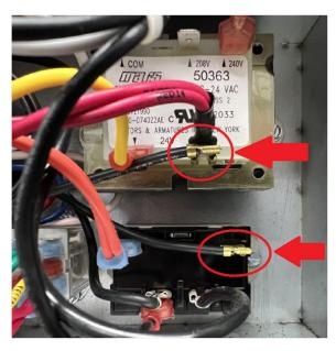
8. Connect both wires by using a jumper wire with alligator clamps or a piece of wire with stripped ends.
