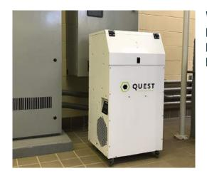
While the industry average remains at only two to three pints, Quest Hi-E Dry dehumidifiers remove up to seven pints of water per kilowatt utilizing a patented revaporator process, designed for efficiency and durability.
