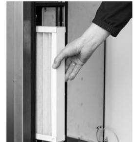
3. Check whether the filter for the control box ventilation system has been inserted:
