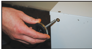
Figure 2: Insert leveling feet in locations.
