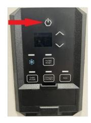
5. Make sure Terminal control light is **NOT** illuminated. Press Terminal Control button to change.
