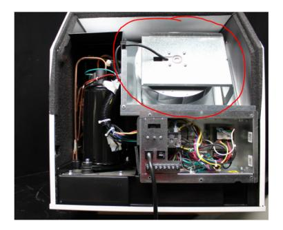
5. Follow the wiring from the fan down toward the compressor area. The wiring plugs into a plastic style connector. Separate that connector. \*Note: this wiring may be wrapped in a black loom to protect it\*
