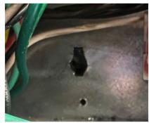
9. Install new capacitor by placing the rear stud through the drilled hole and using plastic nut on the back side of electrical panel to secure.
