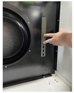
• Inlet ring: Remove fan and bracket to gain access to inlet ring. Place foam tape on edge of inlet ring. Reinstall fan. Turn fan back on to see if noise goes away.
