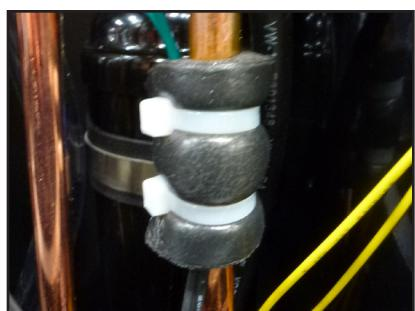
Thermistor attached to the refrigerant line.
