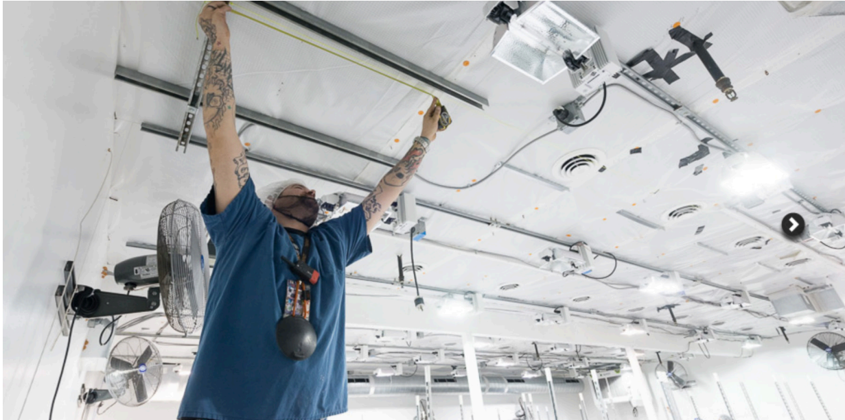
A Grow Op employee prepares to install the Quest 506. Overhead mounting saves space and improves air flow.
