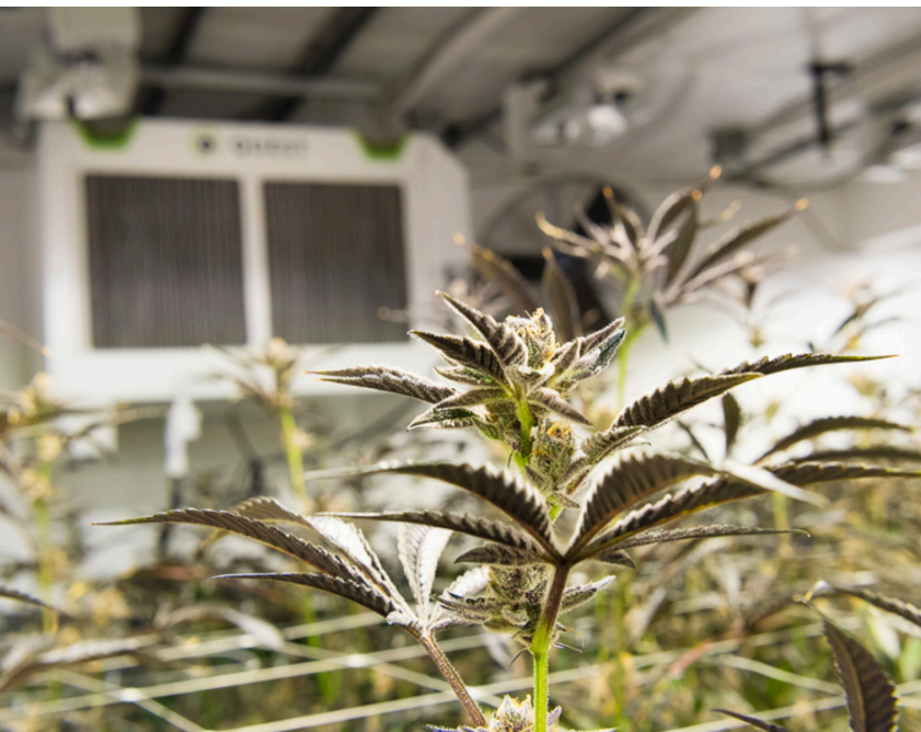
Grow Op Farms used two Quest 506 units (pictured) to stabilize relative humidity levels in Grow Room 3, where it was historically difficult to manage moisture in the air.
