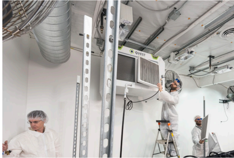
The Quest installation team fine tunes a 506 dehumidifier at Grow Op Farms.
